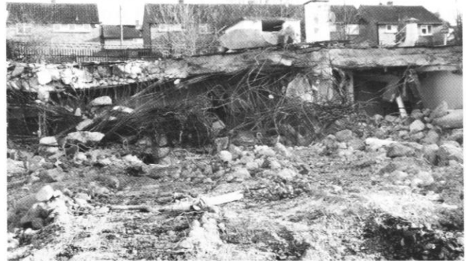
Demolition is underway in mid-November 2012.
